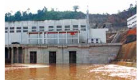
▲ Sluice Gates Closed for Impoundment
