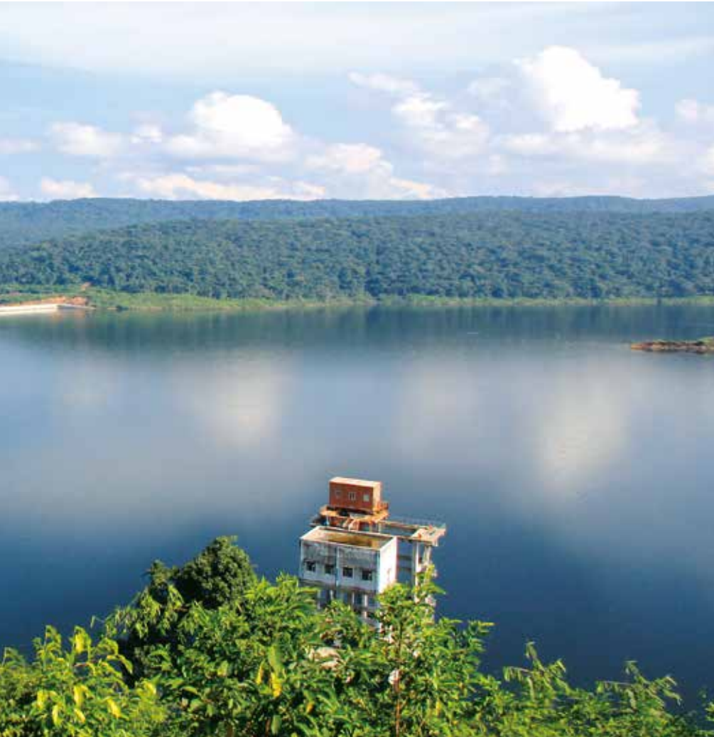
▲ Full View of Cambodian Tatay Hydropower Station
