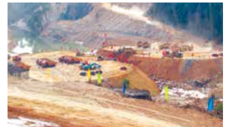
▲ Main Closure Dam
