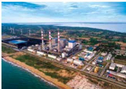
▲ Puttalam Coal Power Project, Sri Lanka
