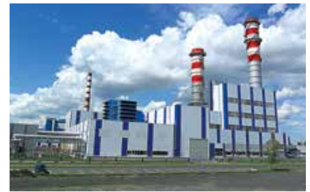
▲ Berezovskaya 400MW Combined Cycle Power Plant, Belarus
